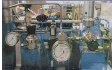
Replacement of a centrifuge instrumentation according to ATEX
