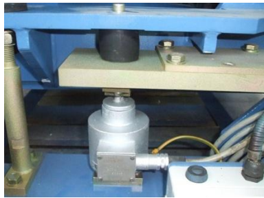
Replacement of a filling control system
